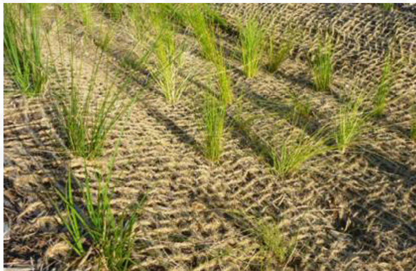
Fig. 4.15: Plantation of vegetation cover and brush wood or coir netting on the slopes of mountain.
