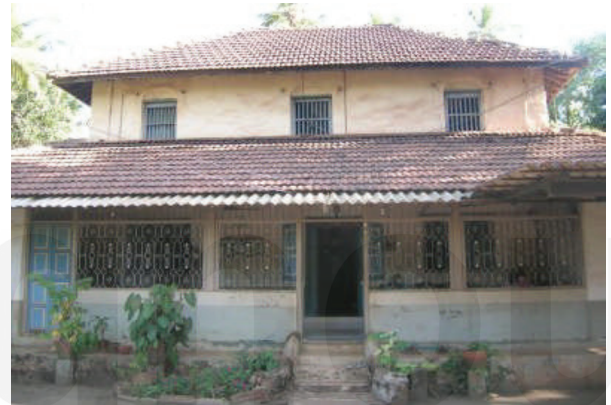
Fig. 14.7: Brick and Mud Slabs House.
